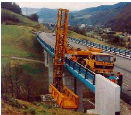
Figure 5: Inspection using a temporary gangway
