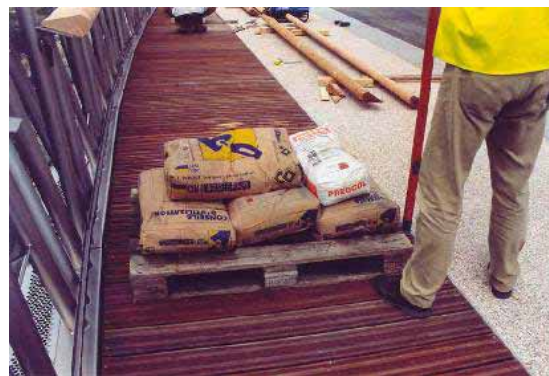
Figure 2: Placing a load on a pavement.
