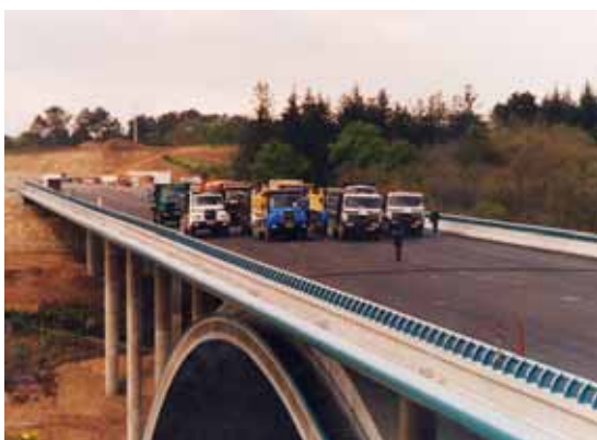
Figure 12: Loading of an arch bridge.
