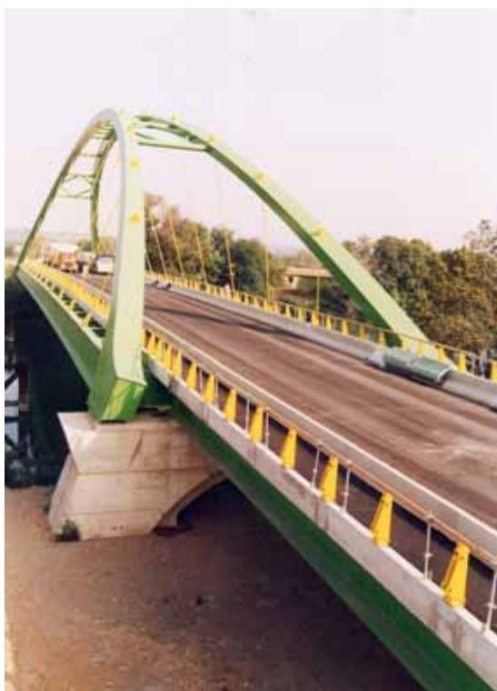
Figure 9: Loading test on a bow-string bridge
