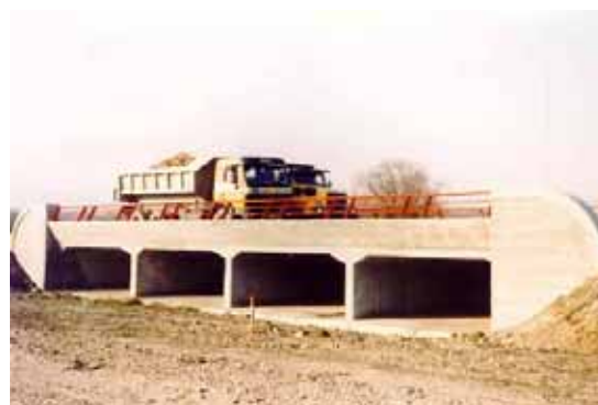
Figure 10: Central loading of a multiple span frame
