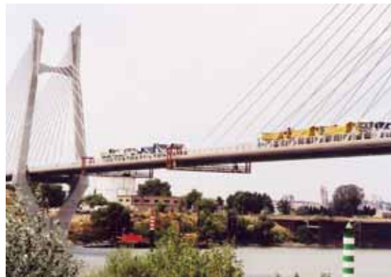
Figure 11: Test loads on a cable-stayed bridge
