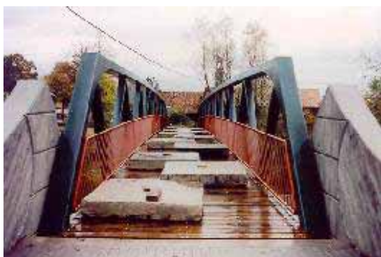
Figure 3: Static tests on a footbridge.
