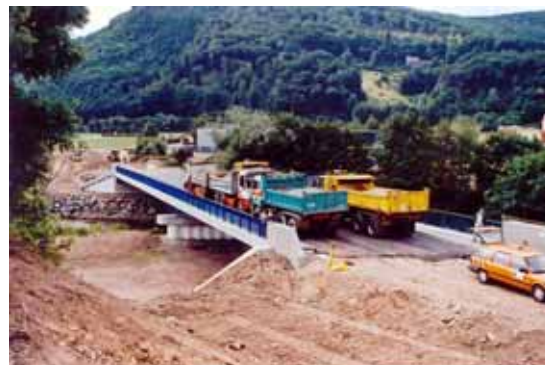
Figure 1: Loading the first span of a slab bridge.
