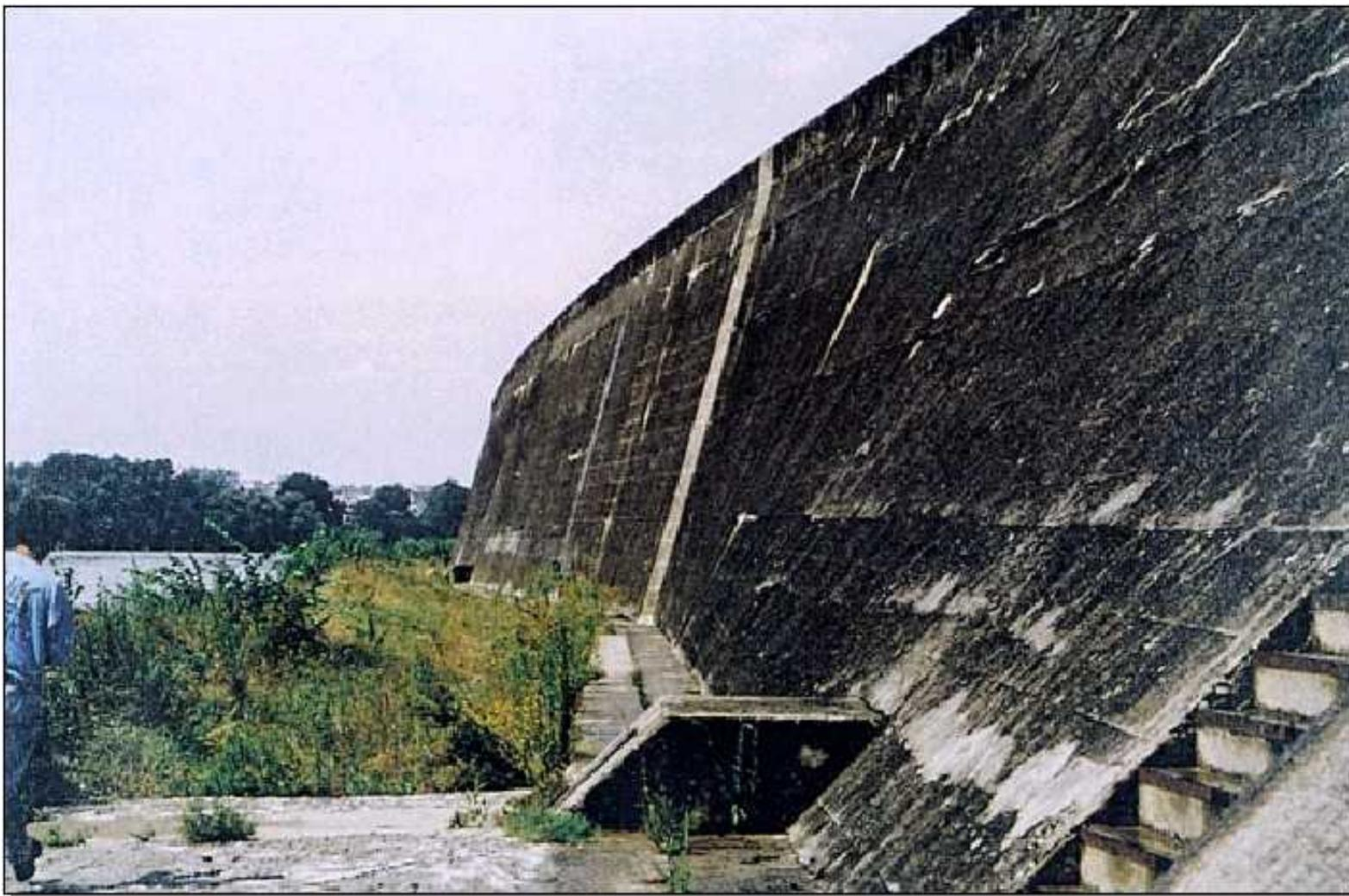
*Mur poids en béton*
