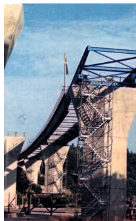
Figure 51 : Lancement ossature
