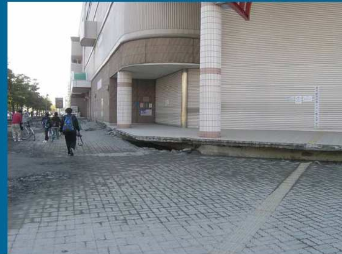
Differential subsidence around pile-supported building and disconnection of lifeline (Urayasu City)
