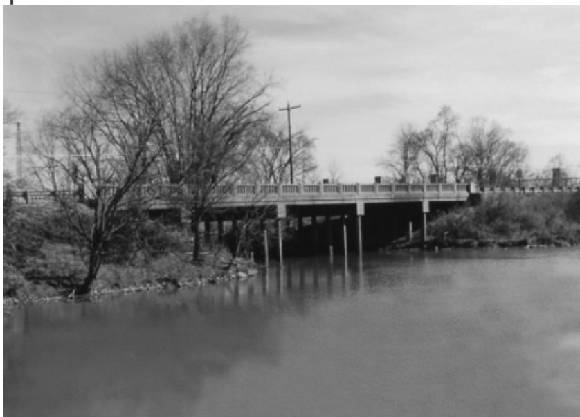
SR 7 Teens Run Bridge at Eureka in southeastern Ohio
