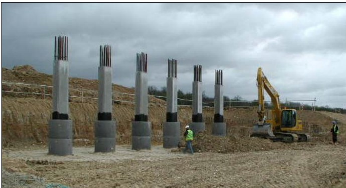
(Photo by courtesy of Mott MacDonald)
