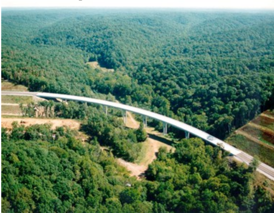
State Route 50 - Bridge over Happy Hollow Creek – Tennessee – 1175feet long (358 m)
