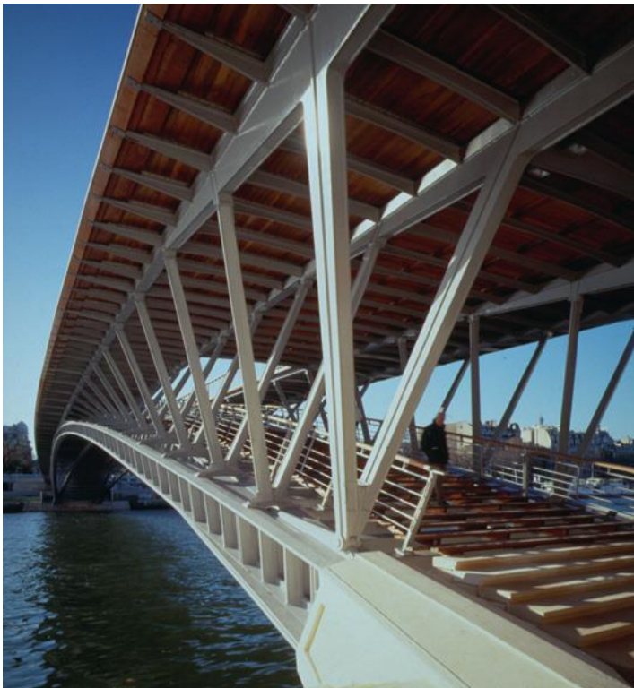
Photo A.4.6 - Passerelle Solferino / Solferino footbridge
