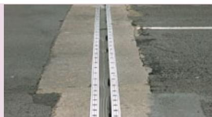
*Ouverture excessive du joint*
