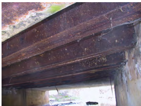
Illustration 82 : Corrosion
