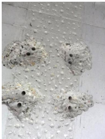
Percements / bouchardage
